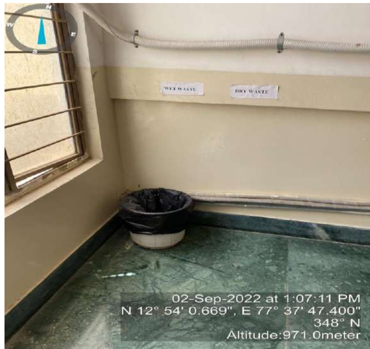
Dustbin in second floor Staircase
